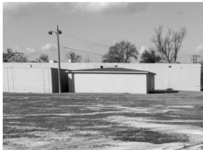
5 Logistics Yard/Storage Building
