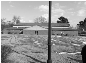
2 Athletic Facilities Complex
